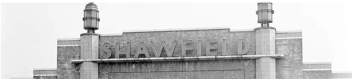
Shawfield Stadium Gates (Glasgow), 1937 (© Glasgow City Archives)
