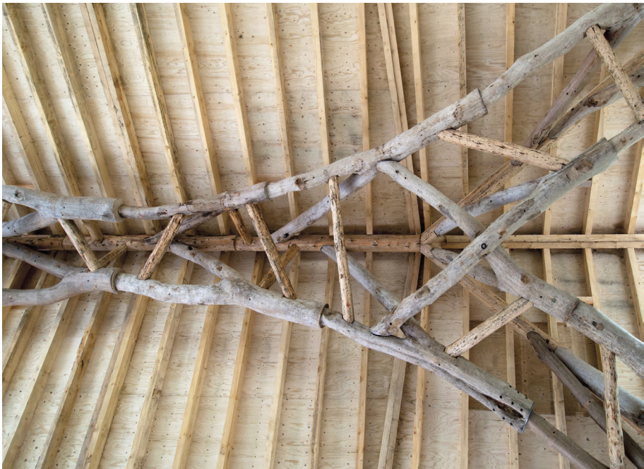
Fig.15- Vue proche de dessous, Wood Chip Barn, AA School Design + Make
