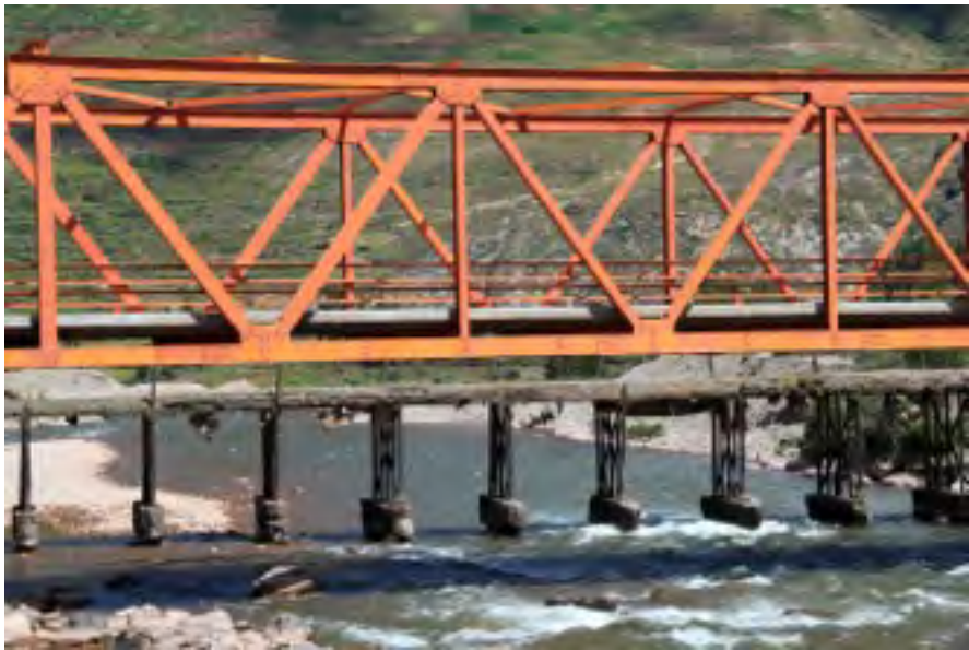
8-1, Combapata, pont contemporain
